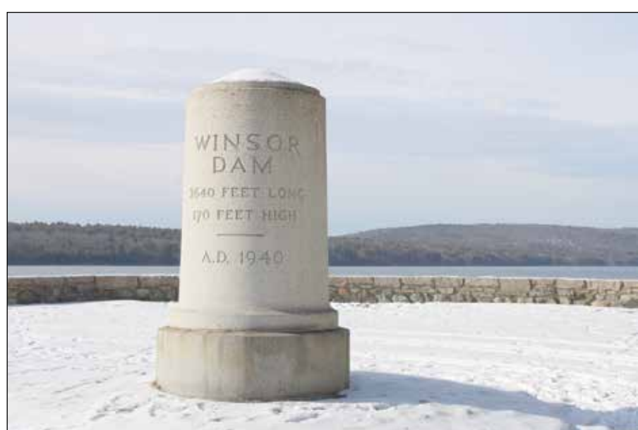
This marker is located at one end of the Winsor Dam, which spans 2,640 feet and is 170 feet high. This dam is the primary impoundment structure for the Quabbin Reservoir.
