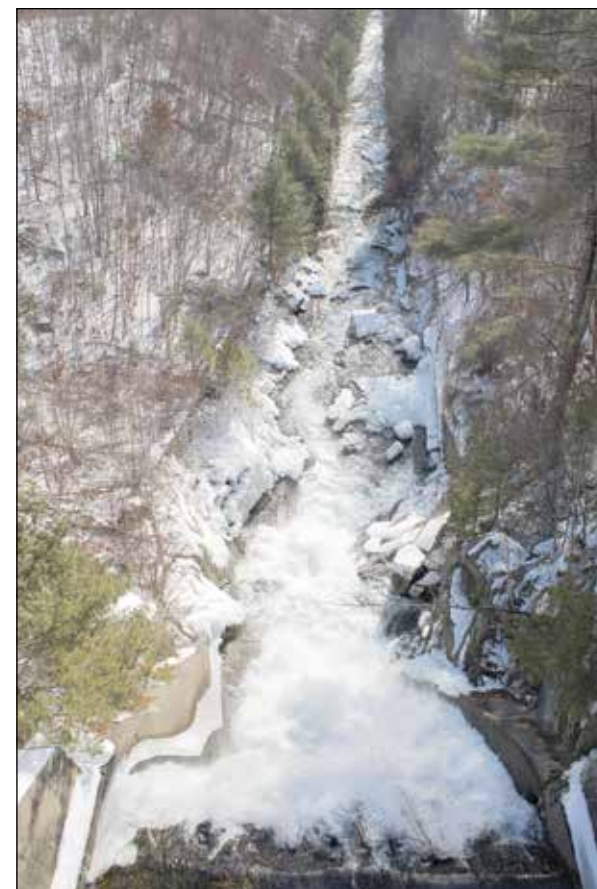
The lower spillway creates a waterfall, and only releases water when the Quabbin Reservoir is at or near capacity.
