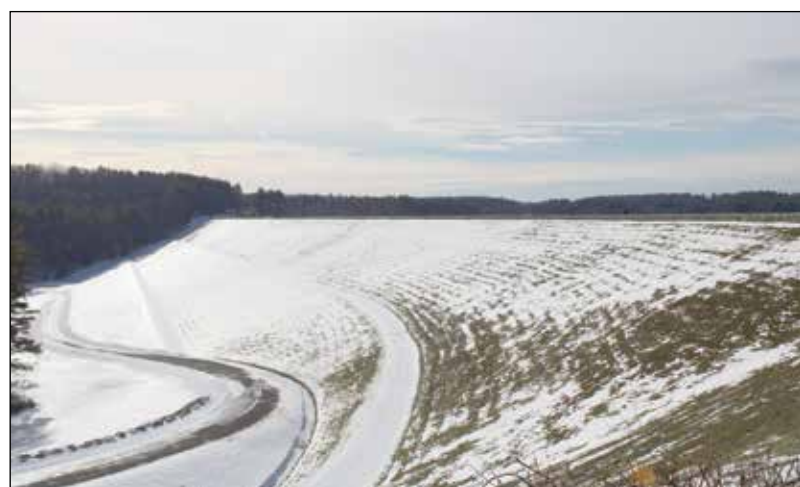
There are 40 caissons buried under this impoundment.
