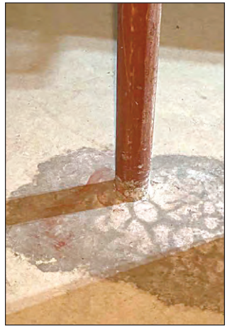
Ground water making its way in through the cracks in the foundation.
